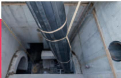
FlexiFlow gates can be retrofitted into existing systems and installed through manholes, minimizing disruption.
