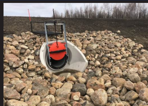
Sluice Gates/Tideflex Valves.
