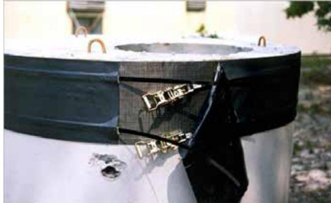
1. Sweep or brush external portion of the joint to insure foreign materials do not interfere with the direct contact between the mastic sealer and the joint to be sealed. Align the collar directly over the joint to where the straps close over the top of the pipe. Remove the protective plastic film, exposing the mastic side to the joint. Wrap the exposed mastic around the joint.
