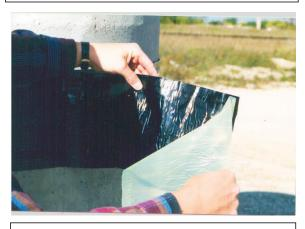
9. Remove the protective plastic film from the back of the closing flap.
