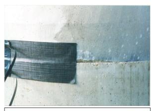
3. Place the exposed mastic side of the wrap against the joint making sure to center the seal over the joint.
