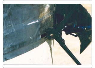
8. Use Crimper Tool to crimp the clip and lock the band in place. Break off the excess band next to the clip by moving the Tensioning Tool back and forth.
