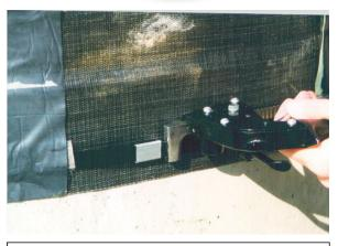
7. Thread the top band through the Tensioning Tool and snug the pusher bar against the clip. Squeeze the handles to tighten the band as much as possible.
