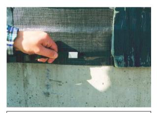
6. Thread the other end of the band through the clip on top of the band end.
