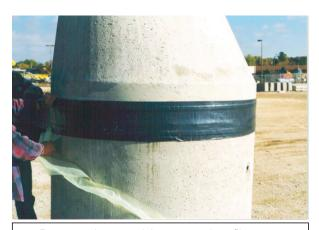
4. Remove the remaining protective film as you continue to place the wrap (keeping it centered on the joint) until the entire joint is wrapped and the ends overlap.
