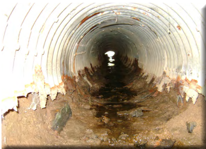
Complete loss of pipe bottom/invert
