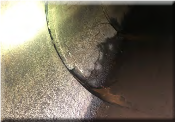
Misaligned joint with voids
