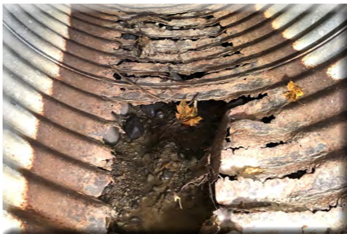
Invert rusting and voids underneath
